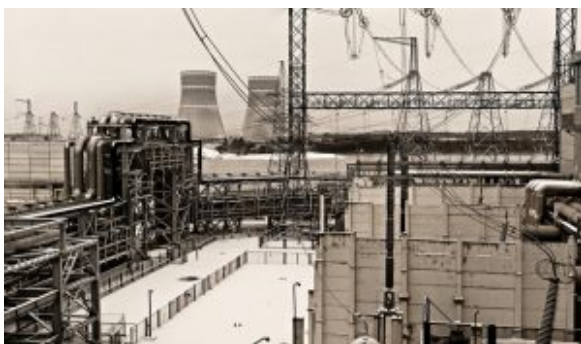
A nuclear power plant under construction (dreamstime)
