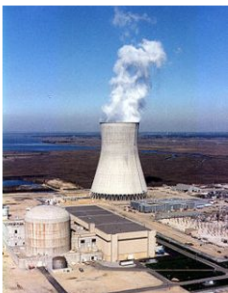
Hope Creek nuclear plant in New Jersey
