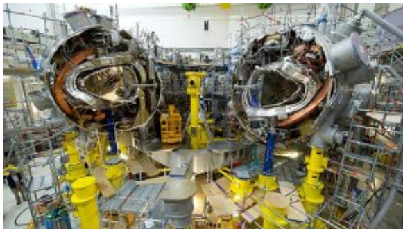
The Wendelstein Stellerator
