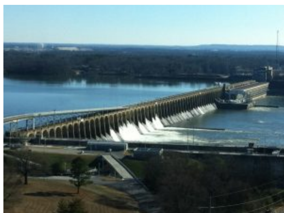
Alabama's Wilson Dam, product of FDR's major infrastructure drive.
